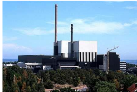
The Oskarshamn 1 and 2 nuclear power reactors
